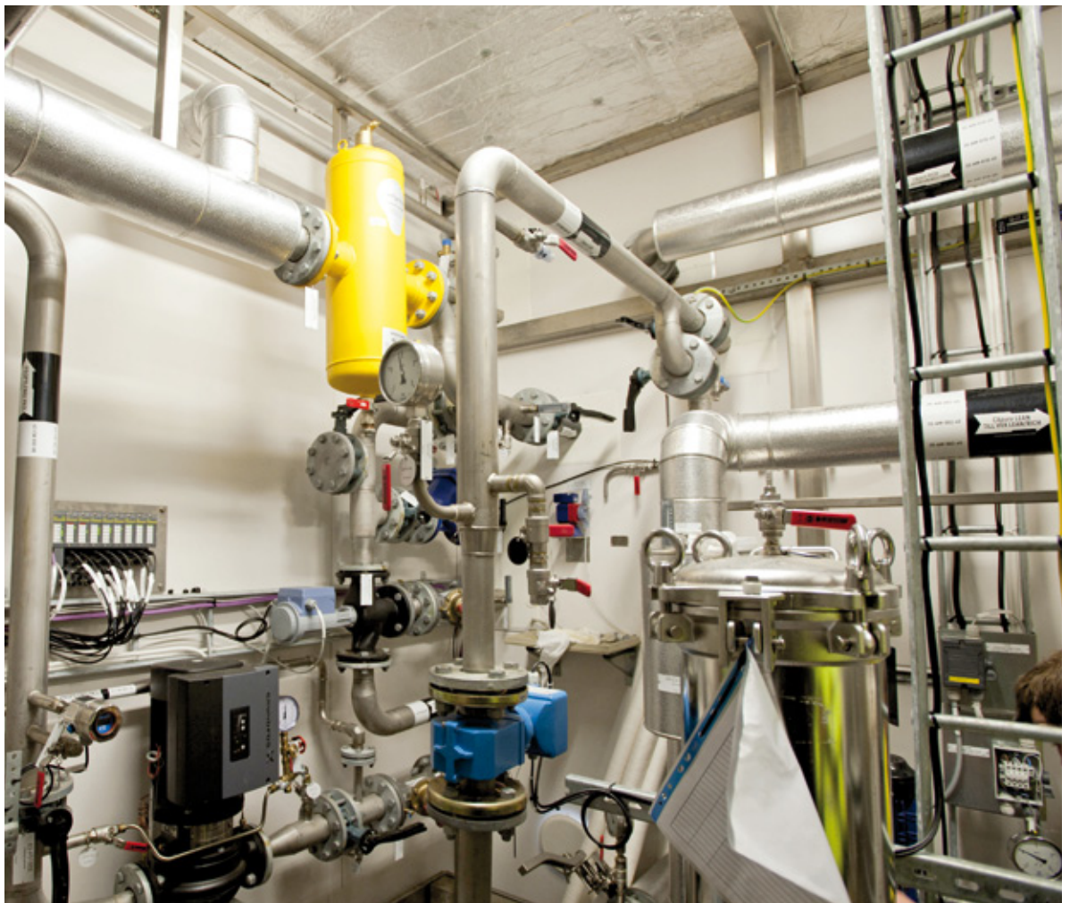
In the hazardous CApure room the BL67 is connecting all sensors to the Profibus
