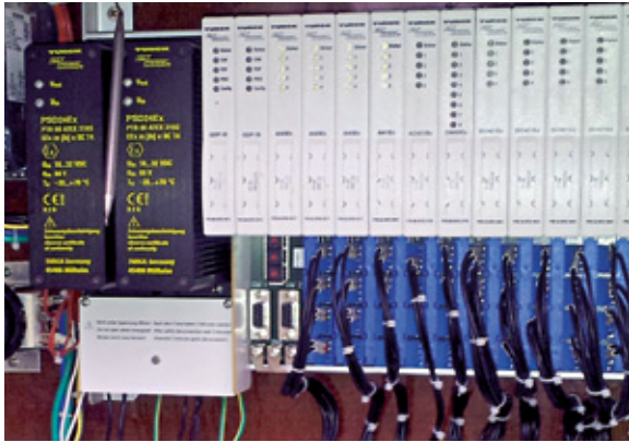
Other modules can be added to excom if field devices need to be retrofitted
